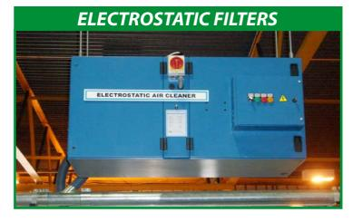
These self-contained Filter Units maybe installed either freehanging or ducted. Removing almost all airborne particulate contaminants, wet or dry, makes these units ideal for many applications, such as;
