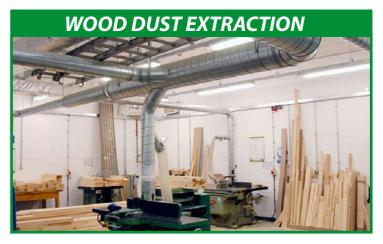
Our Wood Dust Extraction Systems offer an ideal way of removing wood waste before it becomes a health issue. Whether it is a single machine or a complete workshop, we design the system individually to meet all of your requirements.
