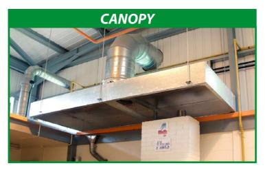
Canopies can extract fumes or gases from a wide general area, where access is not always possible, eg. CNC cutting table or a robotic welder. They are also ideal above cookers etc. in a school or college environment. Custom made to your individual requirements with a high quality galvanised finish.
